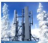
**Wireless DAS** keeps 5G signals in native analog “radio” form as they go up to, and down from the antenna, reducing costs and damage.
